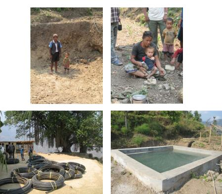
(Upper left:) The pit dug for the tank on land donated by a local landowner. (Upper right:) Community input. Rock breaking for concrete -with immaculately painted finger nails. (Lower left:) Over a mile of transfer and distribution pipe carried up to 1315 meters (over 4,000 feet) by porters. (Lower right:) The finished distibution tank.
